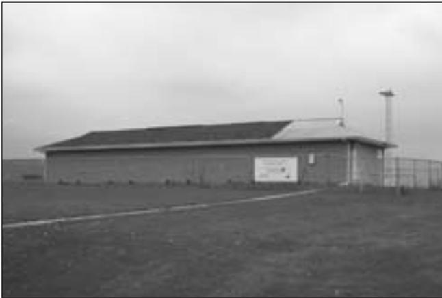
Figure 7 — Bill Rose's shingle temperature data are collected at a test building in Champaign, Illinois. The research building has 10 bays, each 8 ft wide by 20 ft deep. On the roofs of the eight center bays are dozens of temperature probes wired to data loggers. The roofs over the two end bays are not part of the study.
